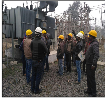
Substation site visit by the participants
