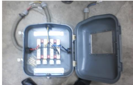
Three phase 3 way Bus Bar
