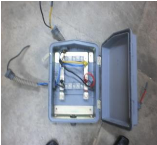
Single Phase 2 way Bus Bar
