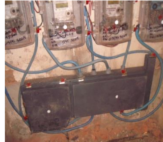
Three phase 8 way Bus Bar
